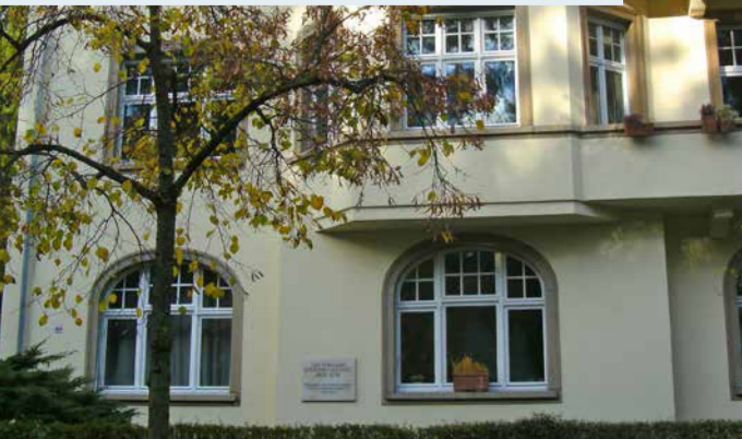
49. Residence of Prof. Husserl, Lorettostraße 40
